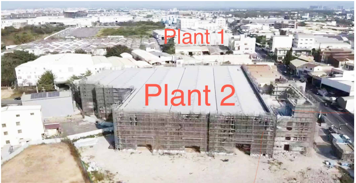
New plants under construction
