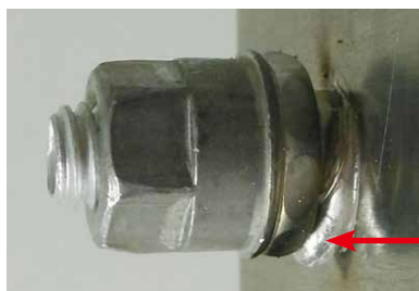
Graphic 3. Hot aluminum fillet can drip during welding process due to gravity, shown at 90 degrees.
