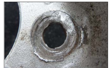
Fig. 2. Red rust and white corrosion product
